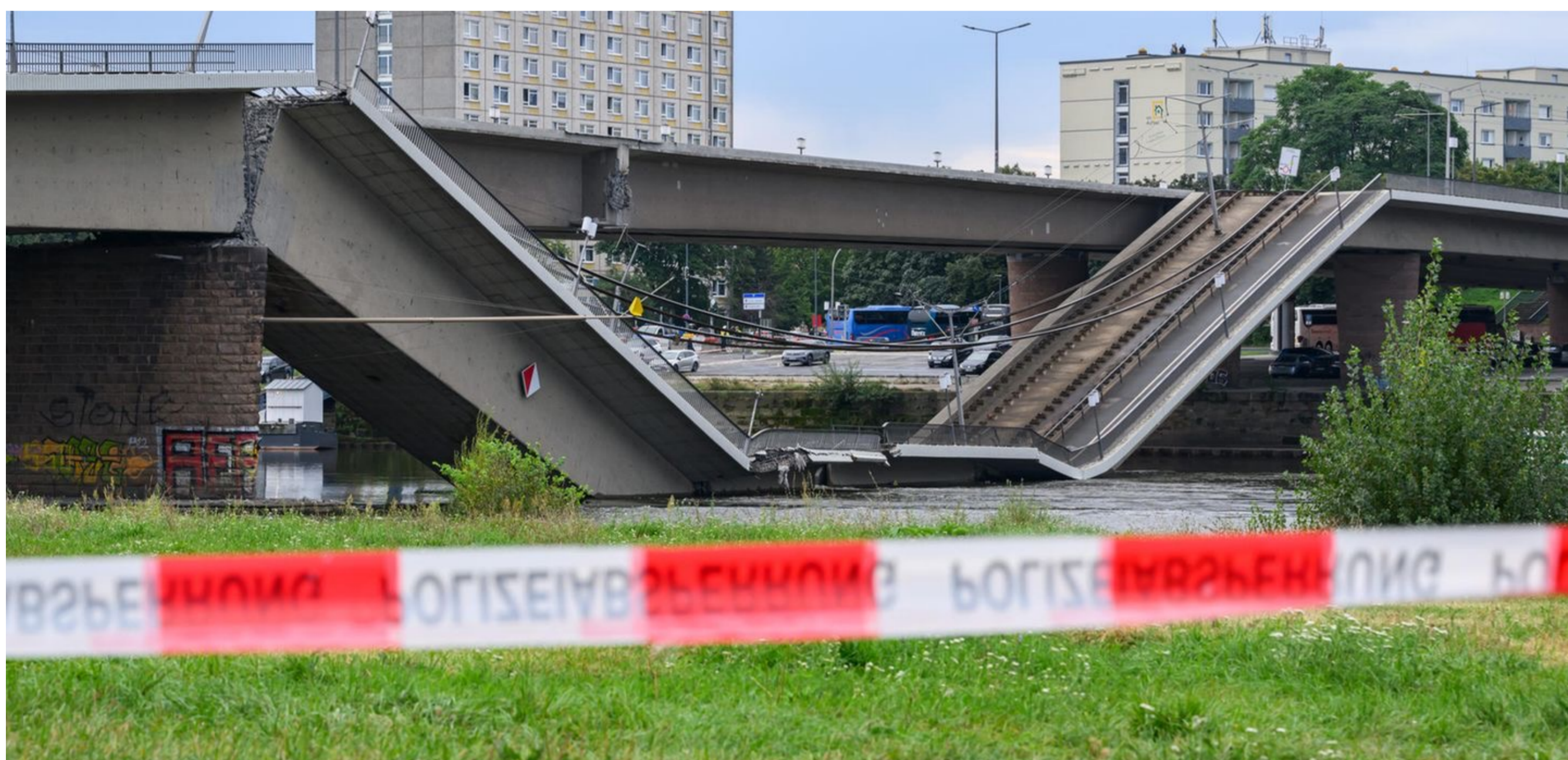
FIGURE 1. Probability of failure: TOO LARGE! Collapsed Carola-Bridge in Dresden, Germany.
