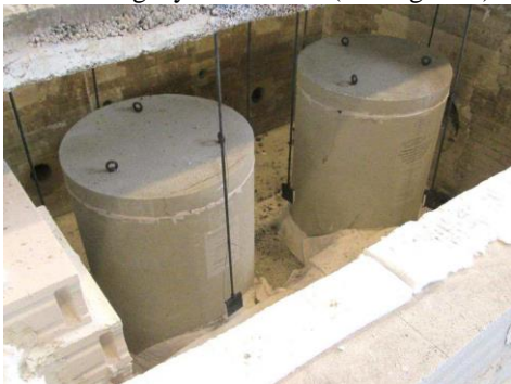
Figure 7. Experimental set-up: final inspection
