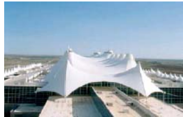
Roof of Denver International Airport
