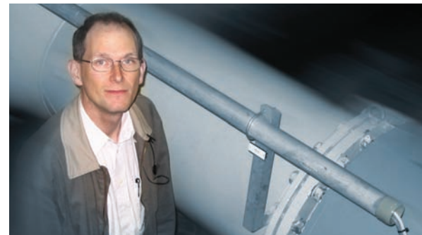
FIGURE 2: Dr. Jan Hofman stands near a flow-meter station at the header of the turbulent ozone reactor at Amsterdam Water Supply. His team positions flow meters such as these at various locations inside its water-treatment facility. Dr. Hofman and other AWS engineers use COMSOL Multiphysics to fill in the gaps between their sparse measurements.
